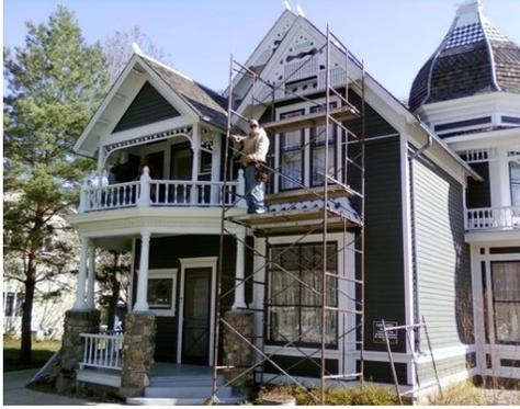
Although the Thompson Crew made the replacement of the Gingerbread 'look' easy, handling the pieces was difficult. Scaffolding, in addition to the ladders on the balconies, was used because of the high and dangerous work. At least three guys
